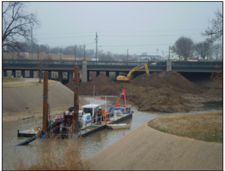
The dredge "Liberty" moves up the creek to remove a large stockpile of material that was pushed "down the creek" with dozers.
